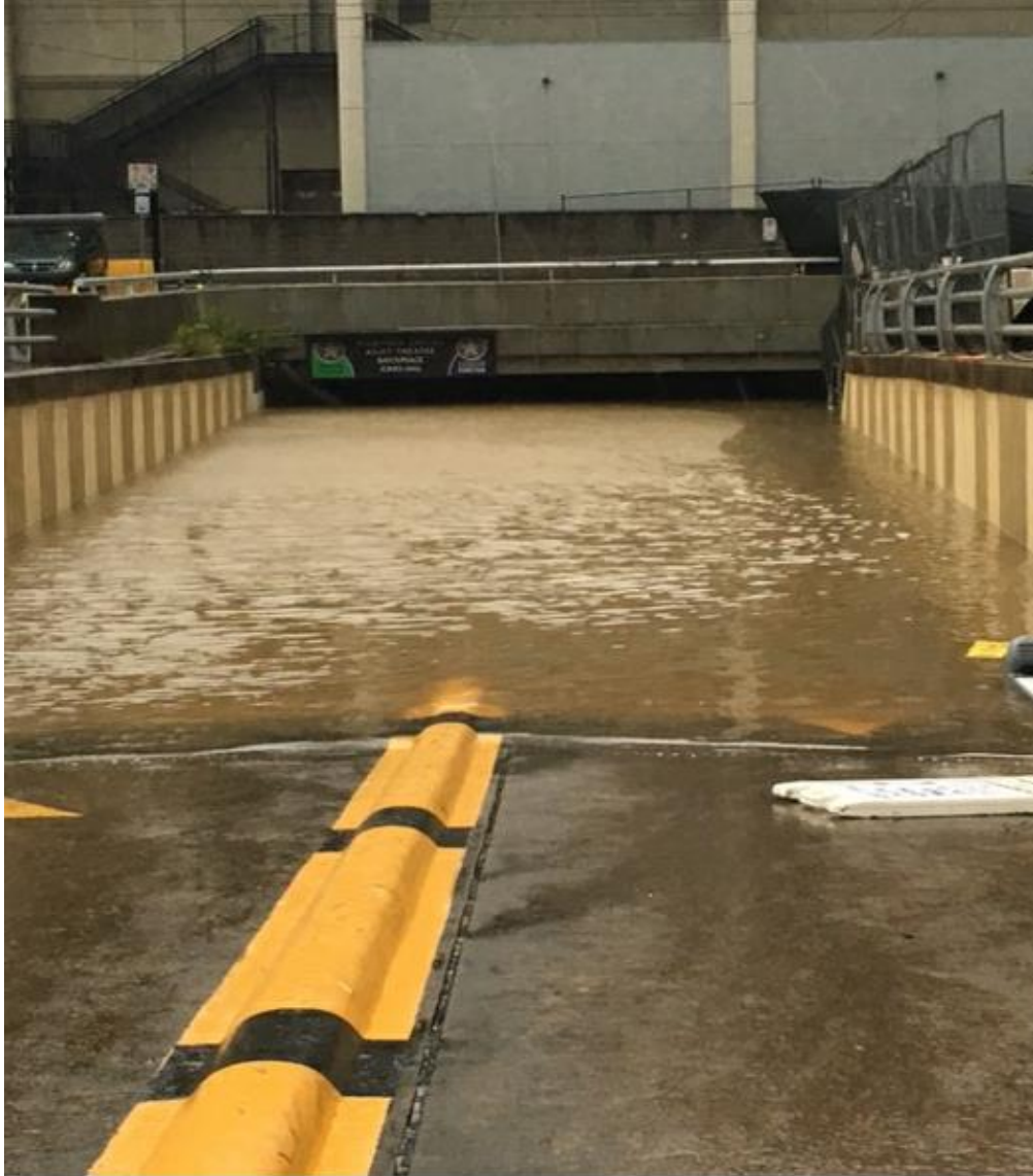
Figure 4. Flooded Garage Entrance on Rusk St. (August 28, 2017)
