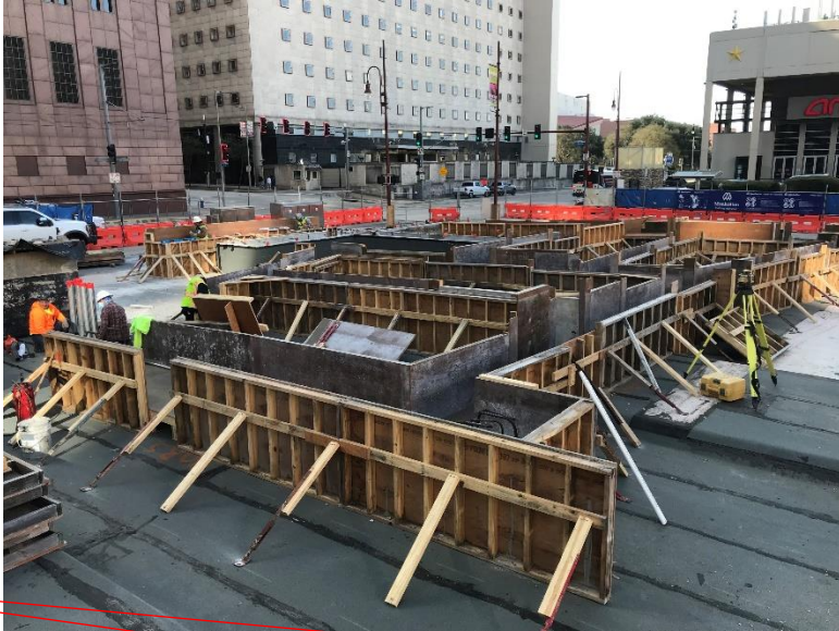
Structural strengthening below for walls above
