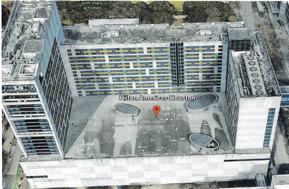
Hilton 6 th Floor Roof Before
