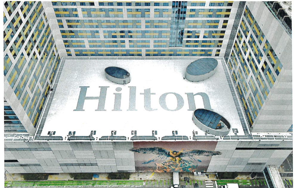
Hilton 6 th Floor Roof After
