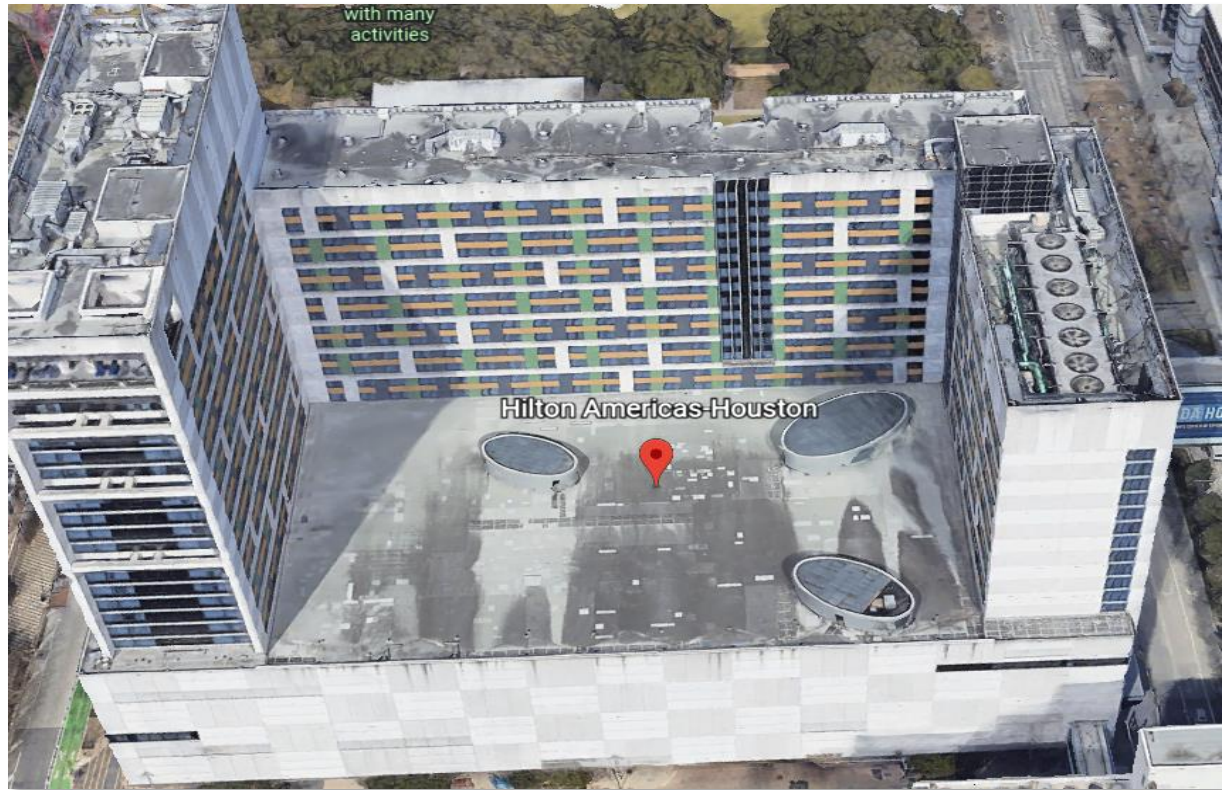
Hilton 6 th Floor Roof Before
