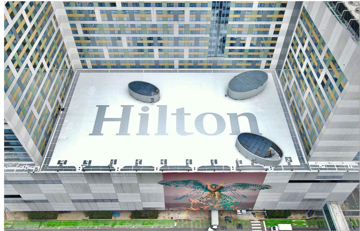
Hilton 6 th Floor Roof After
